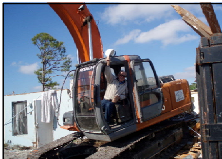
Douglass tearing down the old Safe Space building
